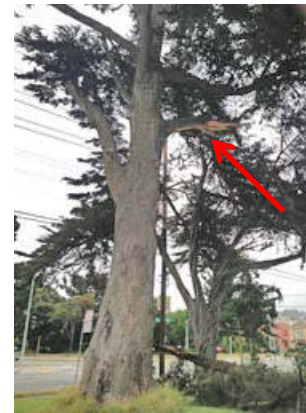
Fig. 2. Many branch failures of Monterey cypress occur along the branch (arrow), commonly associated with heavy end weights and dense crowns.
