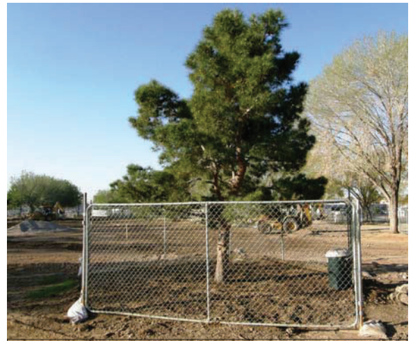
Protecting the root zone of a tree before construction begins is the best way to prevent soil compaction. All photos courtesy: Russ Thompson
