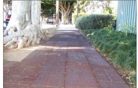
Six years after installation, a rubber sidewalk provides safety while the trees still provide shade. Courtesy: Walter Warriner, Consulting Arborist.
