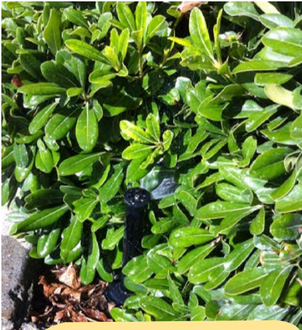
Some of the most common causes of poor irrigation performance are irrigation heads that are broken (top) or obstructed by large shrubs (bottom).
